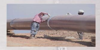
In addition to new construction SPC manufactures products exclusively for large scale pipeline rehabilitation projects. In excess of 300 miles of large diameter pipeline have been recoated with SPC systems. This has included brush / roller application, plural component hand spray and automated line travel spray, both in and out of the ditch. SPC products are employed as repair coating on investigative digs for corrosion and SCC.
