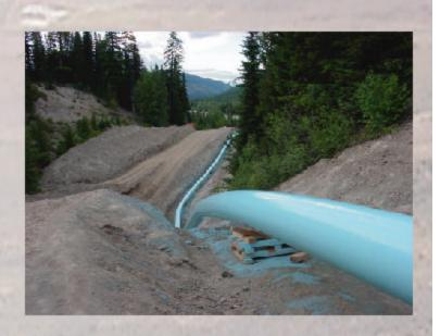
SPC coating systems are rated for in-service temperatures up to 302°F (150°C).
