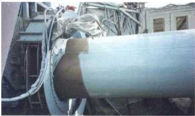
Figure 4. Automated rehabilitation equipment.
