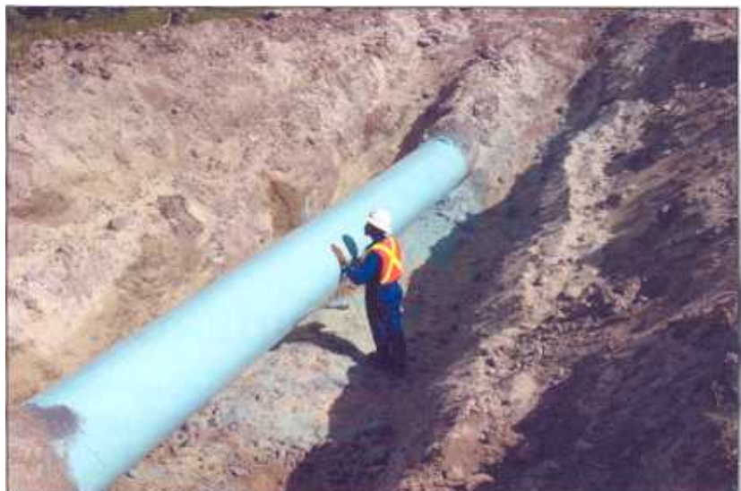
Figure 3. Insitu rehabilitation inspection.
